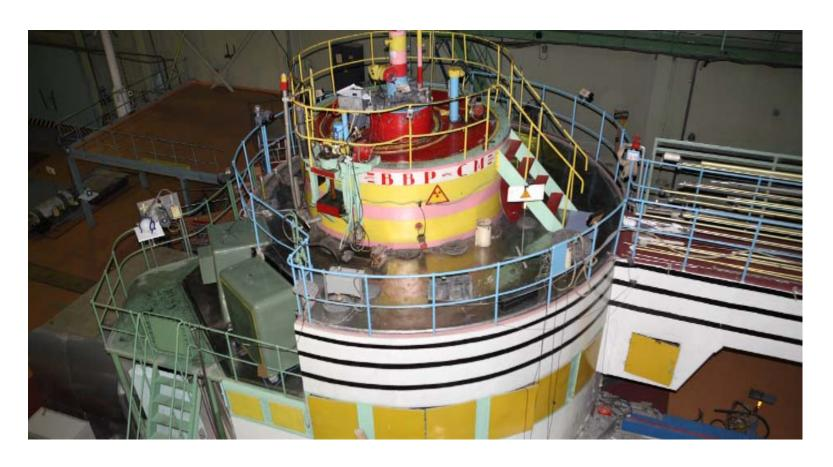
Reactor is used for carrying out researches on nuclear physics, radiation physics, radiation material science, activation analysis, irradiation of minerals, also for radionuclide production.
