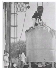
Fifty-ton shipping cask built at Oak Ridge National Laboratory which can transport up to 1 gram of ^{252}\text{Cf} . [58] Large and heavily shielded transport containers are needed to prevent the release of highly radioactive material in case of normal and hypothetical accidents. [57]
