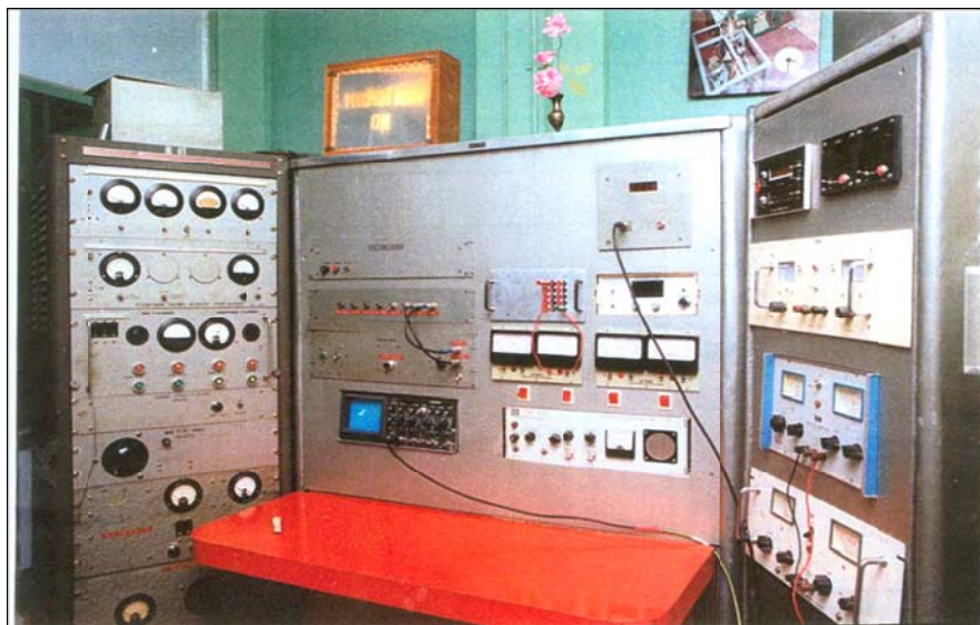
Figure 26: A View of control system of the Race-Track Microtron.
