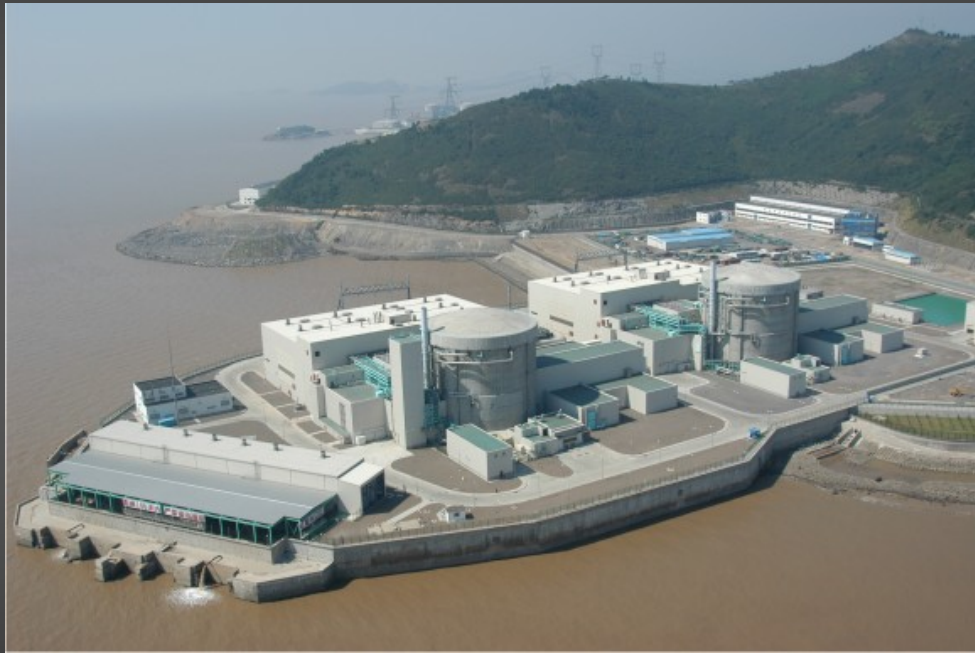
The Candu Qinshan Nuclear Power Plant
